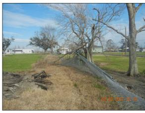
FIGURE 7: VIEW OF DAMAGED SOUTHEAST FENCE NEAR TRAINING BUILDING
