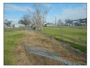
FIGURE 8: VIEW OF DAMAGED SOUTHEAST FENCE NEAR TRAINING BUILDING
