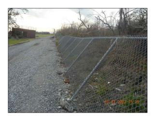
FIGURE 1: VIEW OF LEANING OVER NORTH SIDE FENCE NEAR LIMESTONE ROADWAY
